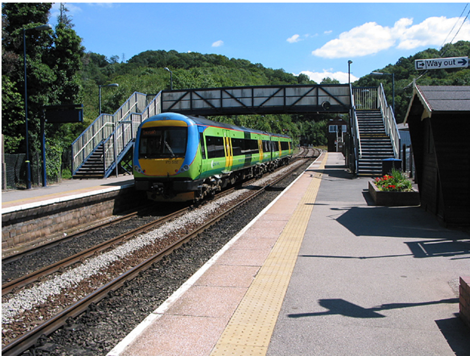
A.3.2 The station as it looks today
